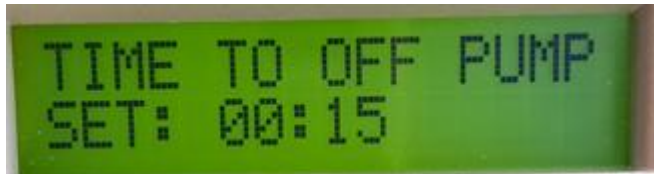
Fig.7. Time to off pump set panel
